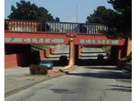
Major circulation infrastructure such as this railroad grade separation on Macdonald Avenue, forms a barrier between the Civic Center and the historic Downtown.
